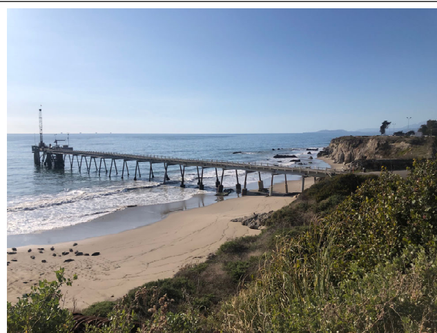
The Casitas Pier was constructed to support offshore oil extractions and the former oil and gas plant, which is in the process of decommissioning.
