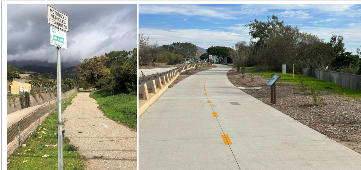
Class I bikeways in the City are provided along Santa Monica Creek (pictured left), along Carpinteria Creek between Carpinteria Avenue and U.S. 101, and parallel to U.S. 101 between Carpinteria Creek and Casitas Pass Road. The new Santa Claus Lane Bikeway (pictured right) was installed in 2024 as part of the U.S. 101 widening project. This concrete path runs adjacent to the Carpinteria Salt Marsh to connect Santa Claus Lane at Sand Point Road to Carpinteria Avenue in the City. Cyclists and pedestrians can now travel from Carpinteria up to the popular Santa Claus Lane shopping and restaurant district and beach, then continue into Summerland.
