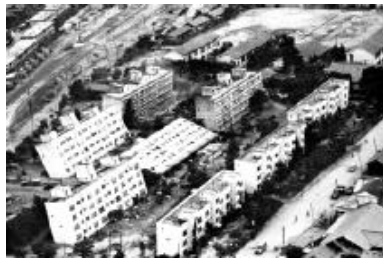
High rise buildings tilted over in Japan due to liquefaction.
