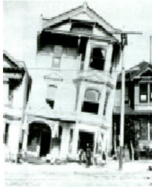
Victorian home tilted by liquefaction.
