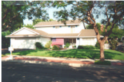
Typical house with prominent garage, but with other elements of the facade dominant.
