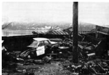
Tsunami damage in Alaska due to 1964 earthquake.
