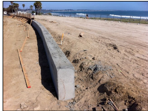
Construction of Parapet Wall
