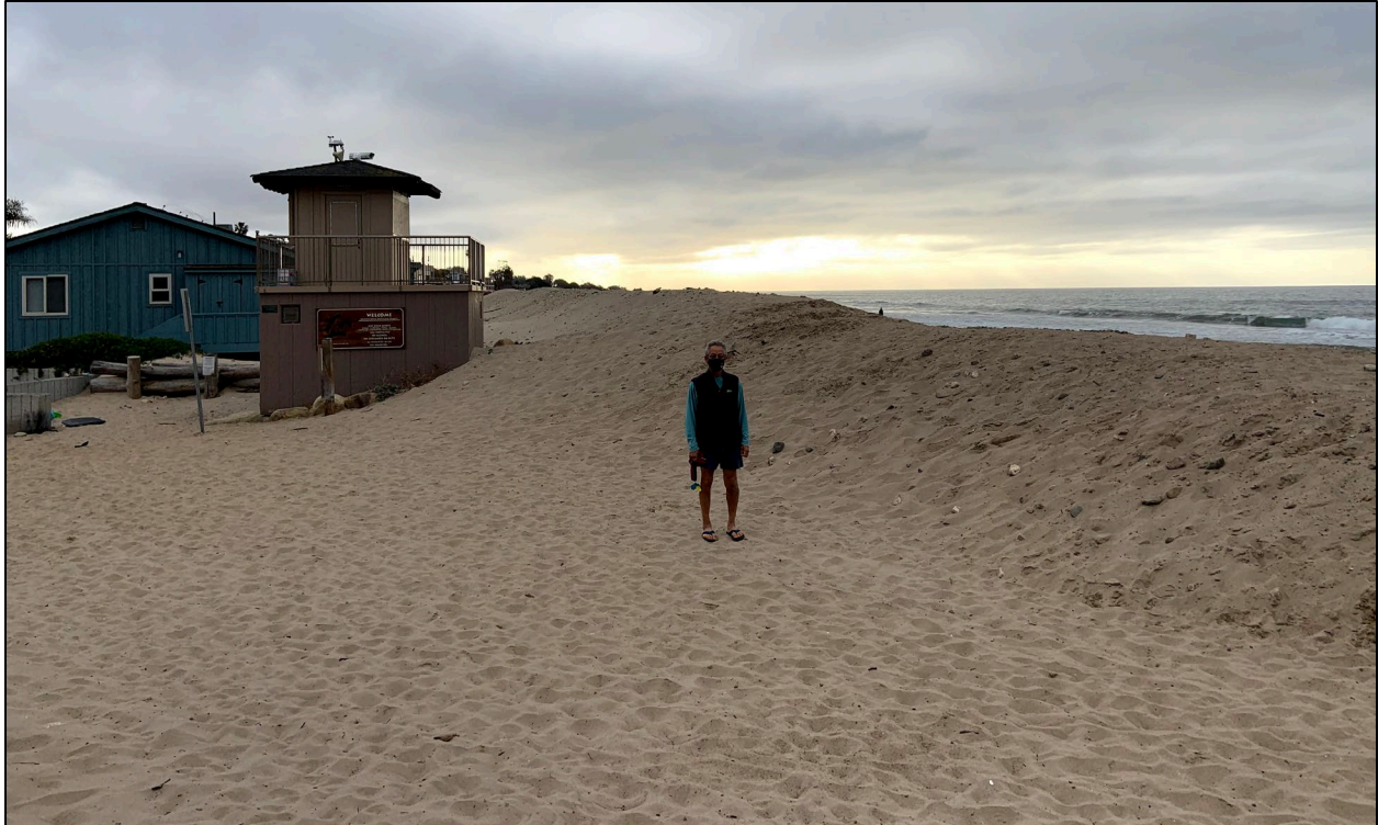
Figure 3.2. City of Carpinteria Winter Dike, North End at Ash Avenue – January 2021, Showing Continuous Alignment Across First Floor Views
