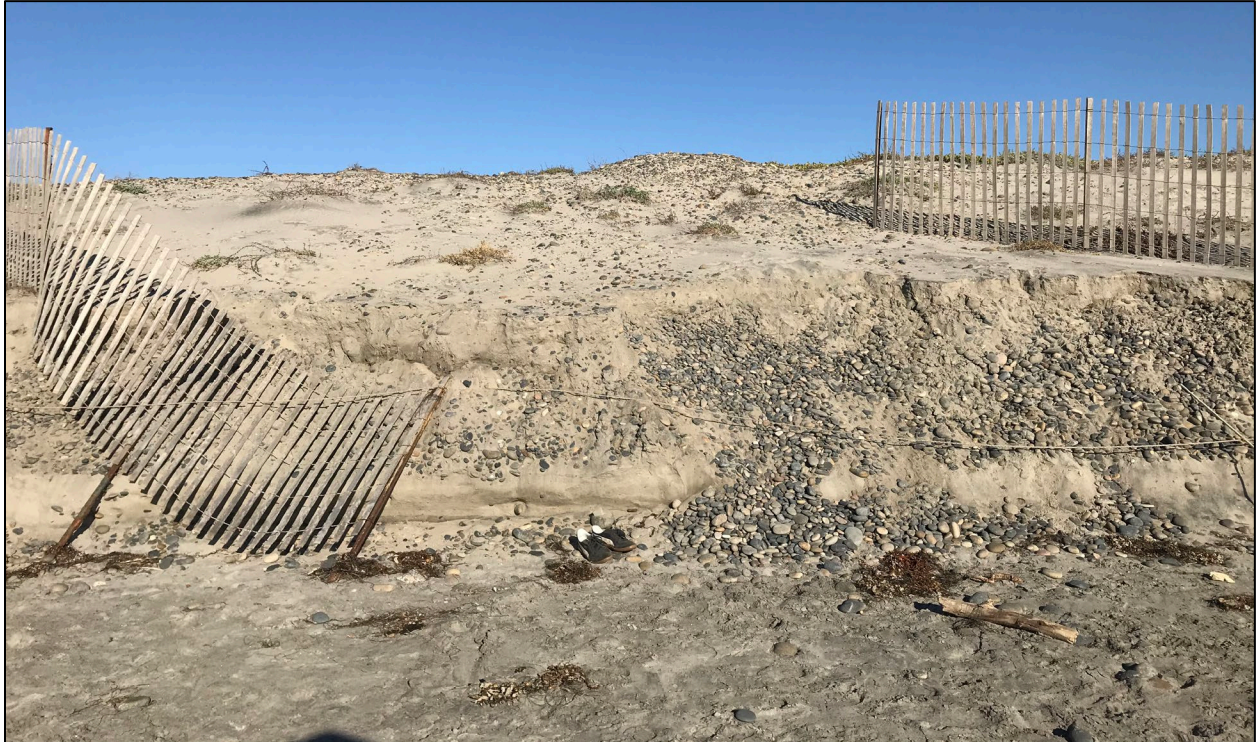
Figure 3.7. Cardiff Living Shoreline, Erosion Exposing Cobble Toe – February 2021
