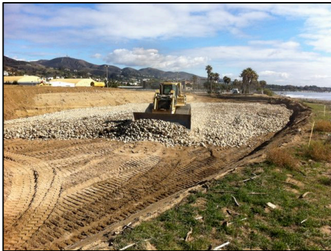
Construction of Cobble Berm
