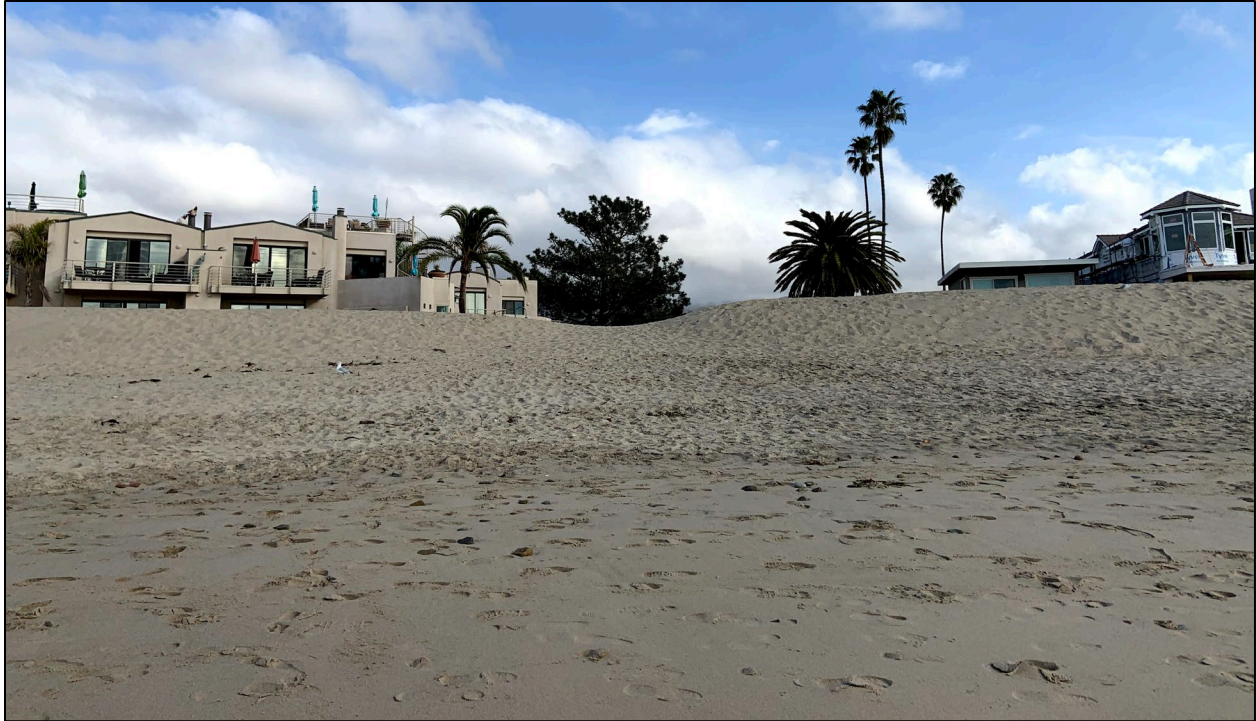
Figure 3.4. City of Carpinteria Winter Dike, Mid-Reach at Elm Avenue January 2021, Showing Modest “Saddle” in the Crest for Access
