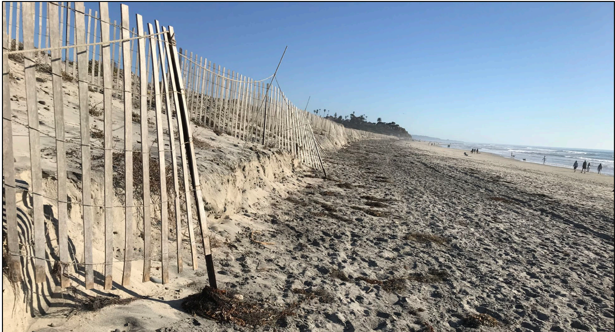
Figure 3.8. Cardiff Living Shoreline, Toe Erosion and Undermining of the Dune Fencing – February 2021
