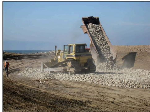
Importing of 6- to 18-inch Diameter Cobble
