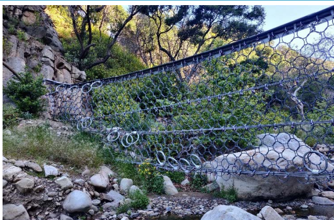
Area debris nets have prevented sediment, sand, and cobble from reaching beaches, and the deposition of this sediment on area beaches has been difficult to facilitate.
