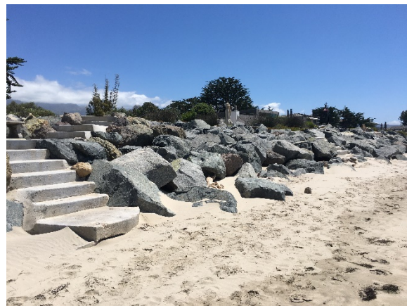
Existing coastal armoring in Reach 1 could reduce feasibility of a living shoreline due to more limited beach widths and increased costs of construction if removal of armoring were required.
