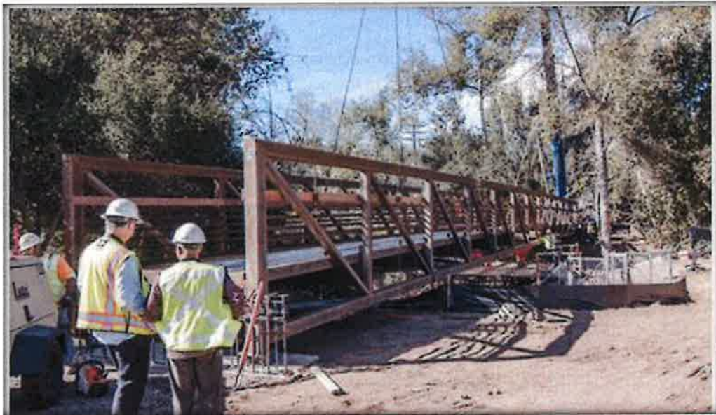
Illustration 2-4 Representative Steel Framed Bike Path Bridge
