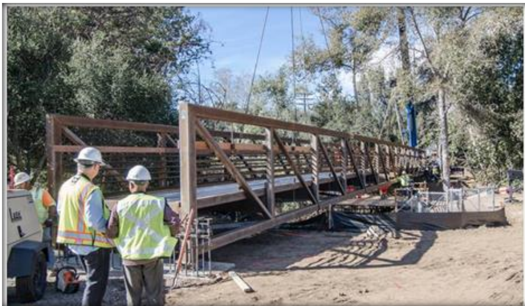
Illustration 4 Representative Steel Framed Bikepath Bridge
