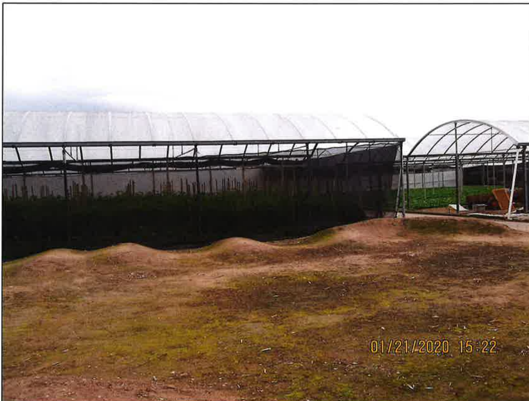
The above greenhouses, located at 1552 Casitas Pass Rd (APN 001-060-040) have a pending permit (19CDP-00000-00058) to utilize these open-sided "mixed light" structures for cultivation of cannabis.
