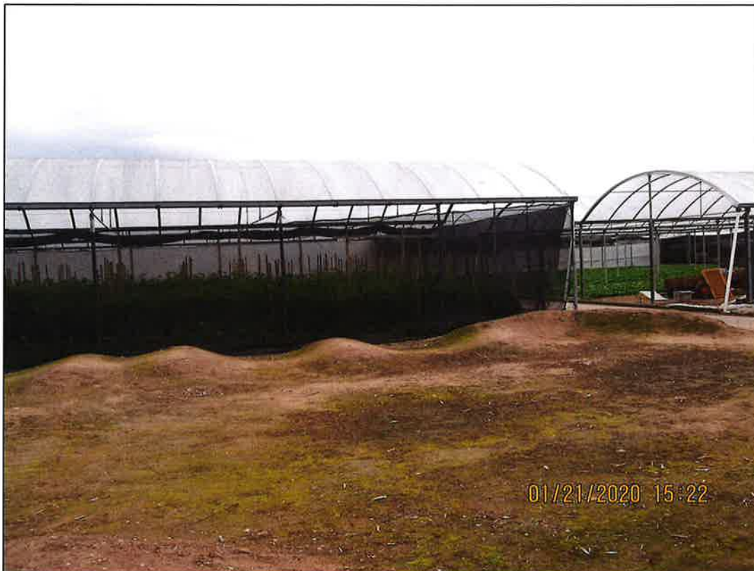
The above greenhouses, located at 1552 Casitas Pass Rd (APN 001-060-040) have a pending permit (19CDP-00000-00058) to utilize these open-sided "mixed light" structures for cultivation of cannabis.
