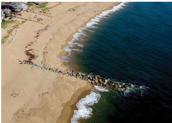
A cross-shore rock revetment has been implemented in Plum Island, Massachusetts, to retain sand and protect vulnerable neighborhoods from beach erosion. Photo Source: City of Newburyport.
