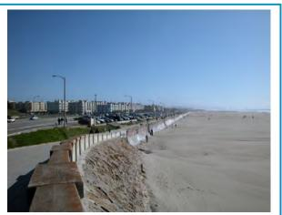
Example of hard shoreline protection. Portions of San Francisco's Ocean Beach is partially armored by a concrete seawall and supplemented with regular beach nourishment.
