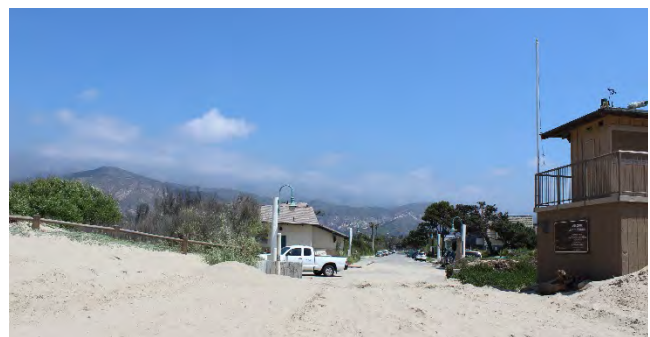
Sand from Carpinteria City Beach abuts Ash Avenue, which serves as a buffer from wave attack and runup damaging and eroding the roadway. With approximately 2 feet of sea level rise, erosion of this sand buffer could result in damage to this roadway, as well as at Linden, Holly, and Elm Avenues, which also terminate at the sandy beach.
