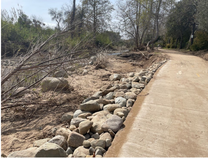
Photo 2. Washed out portion of the creek bank along the bike path
